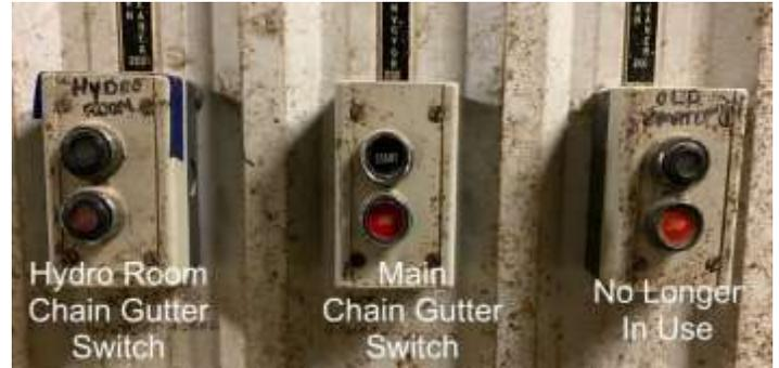
Figure 1: Chain Gutter Controls
