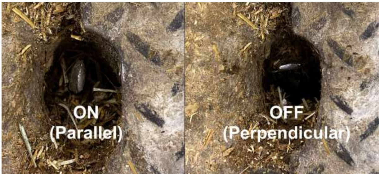
Figure 1: Gutter Valve Position
