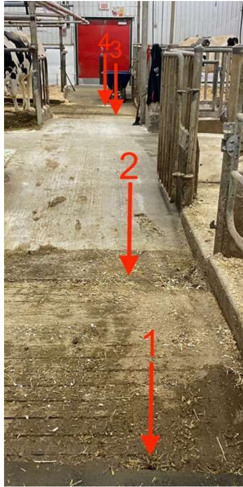
Figure 3: Gutter Valve Location
