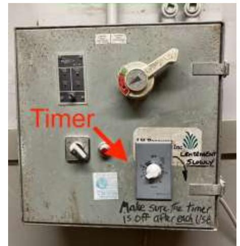
Figure 4: Gutter Control (Pre-pit pump timer)
