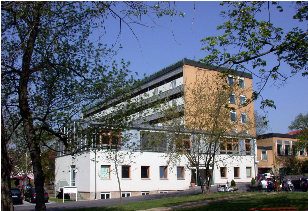
University Children's Hospital, Wuerzburg, Germany
