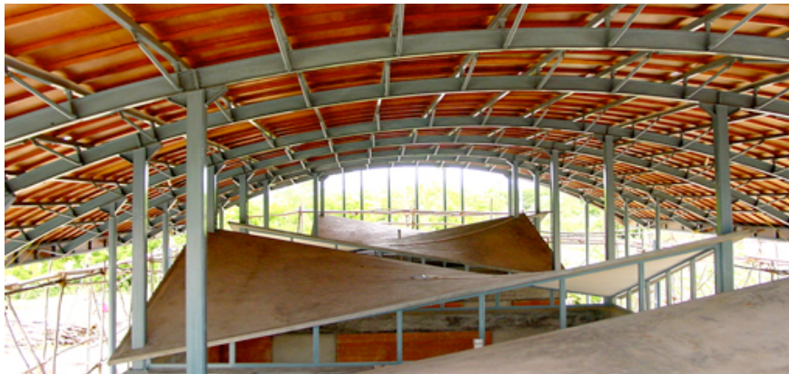
Figure 12 U.S. Pavilion Auroville, Tamil Nadu, India, 2002 A double-roof system that encourages natural ventilation and shedding
