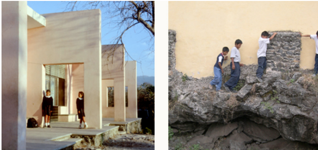
Figure 8 Escuela San Lucas Tejalpa, Morelos, Mexico 1995-1997 (The addition of buttresses on the western courtyard façade interrupts the sun's hot rays and creates a shady loggia in front of the building. ( the Basic Initiative) Source: http://www.basicinitiative.org/programs/global_communities/Escuela_San_Lucas.htm
