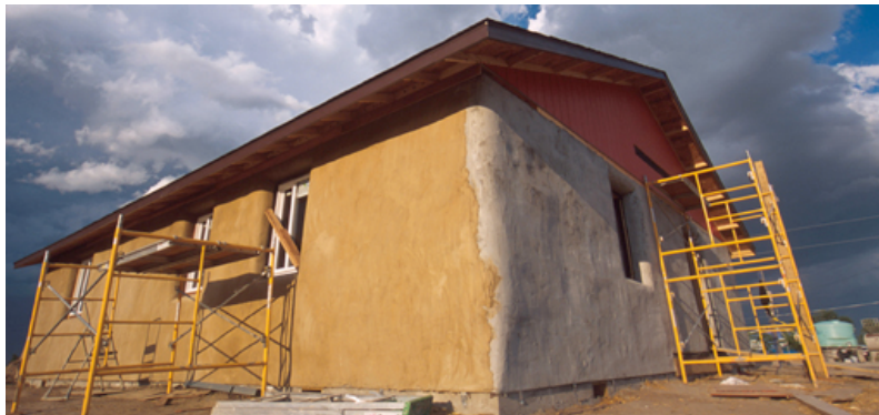
Figure 2 Fast Wolf House Pine Ridge, SD 2000 straw bale house (by the Basic Initiative)
