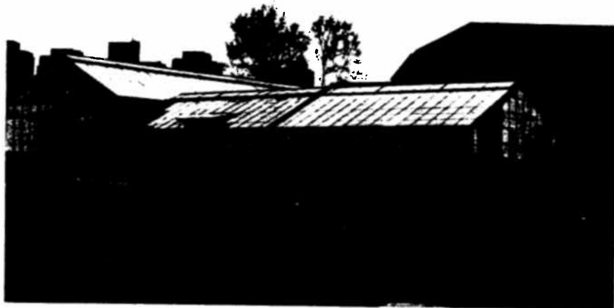
Exterior view along McGregor Avenue.
