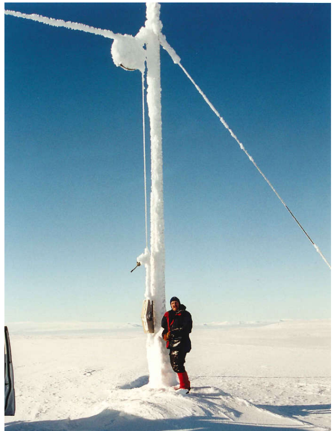
Fig. 4 The first generation of test spans: The conductor goes over a wheel near the top and is connected to a mechanical dynamometer ca. 1,5 m above ground.
