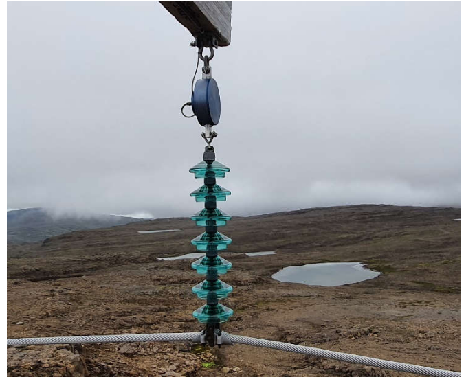
Fig. 7 The old digital tension recorders with built-in amplifiers are used in suspension strings in older 132 kV lines. A cable connects it to a data logger and a GSM sender at the base of the pole.
