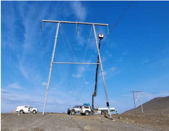
Fig. 11 The measuring device is mounted in a new 220 kV tower.
