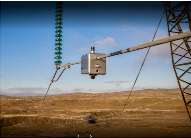
Fig. 15 Device from Laki Power installed on a conductor. Its power source is induced from the conductor.
