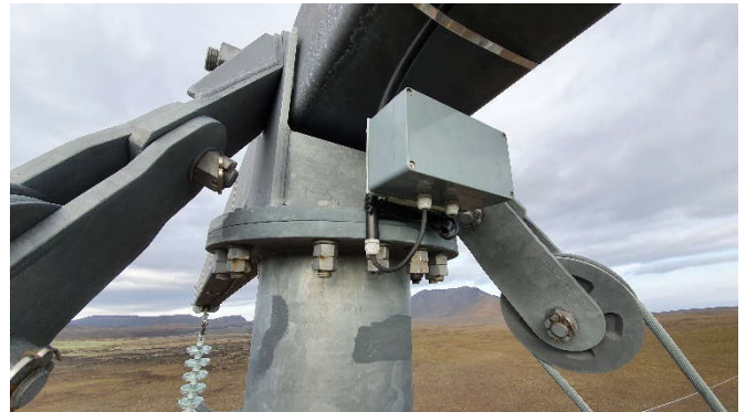
Fig. 13 A box with an amplifier is mounted below the cross-arm.
