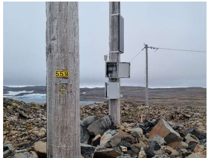
Fig. 8 A box with a GSM sender is mounted on the tower leg with a solar panel above, a battery below and a cable from the measuring device. A digital thermometer is above the box, ca. 2 m above ground. In the background is the old test span at the site, which will be replaced by the measuring site in the operating line.
