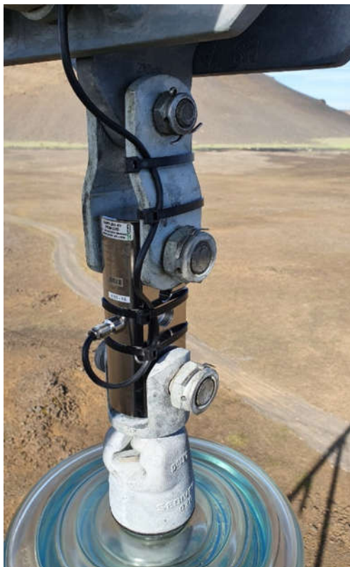
Fig. 12 A load cell in an insulator string in a new 220 kV transmission line. A cable connects it to an amplifier and to a data logger and GSM sender at the base of the tower.
