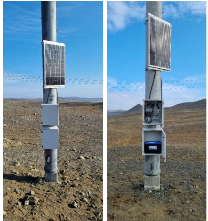
Fig. 14 The GSM sender is mounted on the tower leg with a solar panel above, a battery below and a cable from the amplifier.
