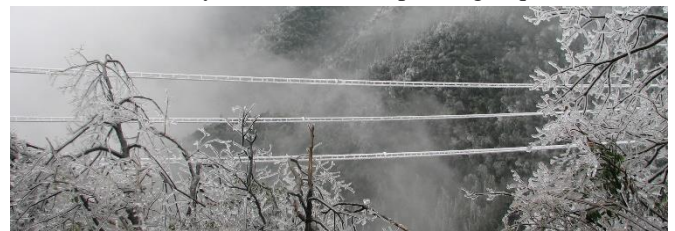
Fig. 3 Iced conductors of the 220 kV line.
