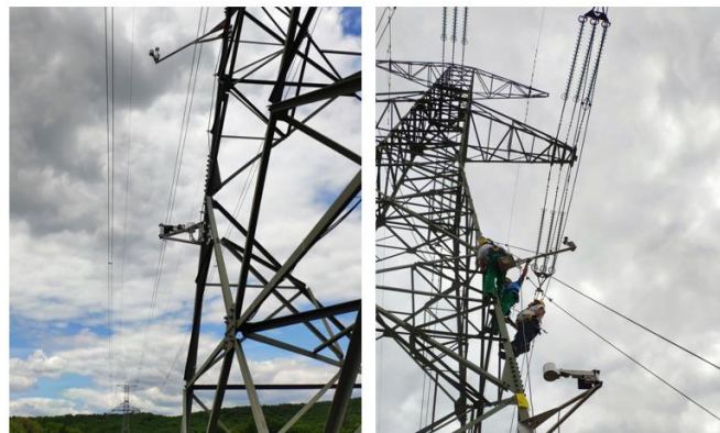
Fig. 3 Weather station installed onto the Göd-Levice 400 kV power line [11].
