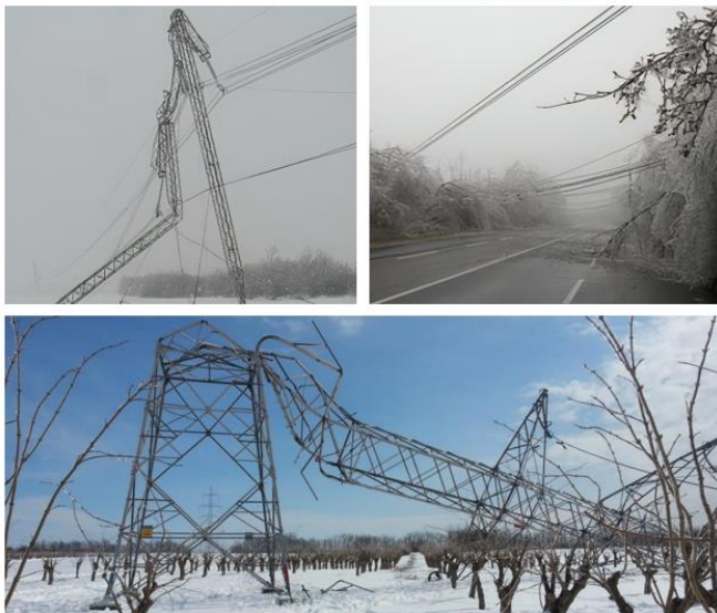
Fig. 1 Collapsed towers and damaged conductors since icing events in Hungary over the last decade [4][5].
