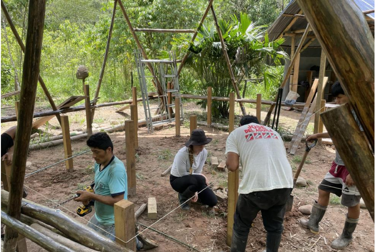
Construction of the main classroom, Schumacher placement, 2022.
