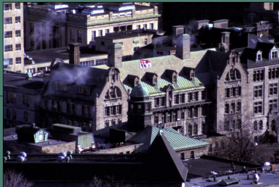
The Macdonald Engineering Building, home of Civil Engineering
