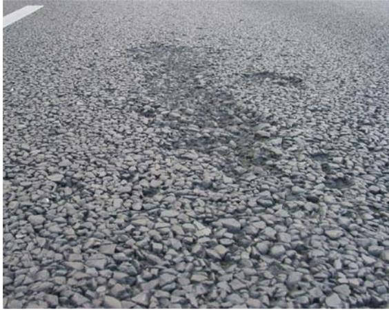
Figure 2: Raveling of the asphaltic wearing surface
