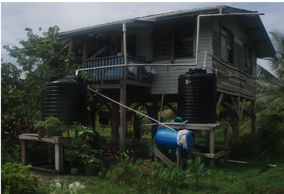
Typical housing in St Cuthbert's, Guyana with rain water harvesting technology.
