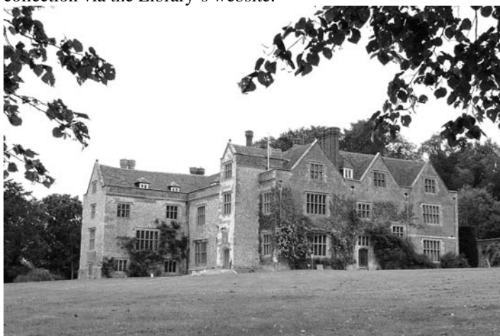
Chawton House Library, showing the south and west fronts. Photographed by Steve Shrimpton (Kind permission from CHL).
