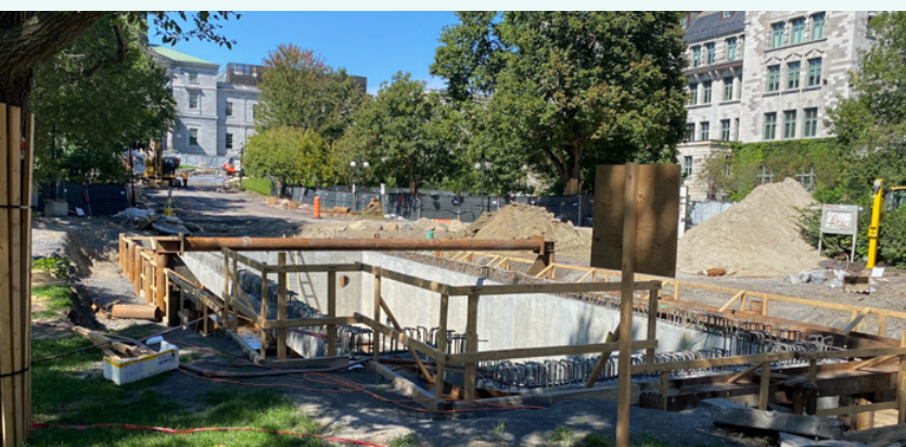
Water retention infrastructure being installed as part of McGill's reconstruction of the upper main road
