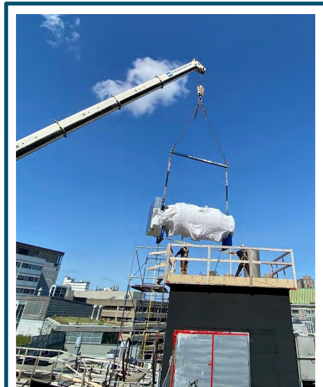
In September 2023, an electric boiler was delivered to the downtown Powerhouse for the Boiler Replacement and Heat Recovery Project.
