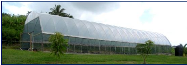
Figure 1. Greenhouse built with local materials in the Parish of St. John
