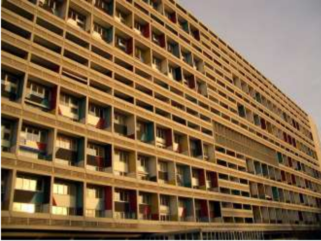
Figure 18 Le Corbusier Unite habitation, Marseille
