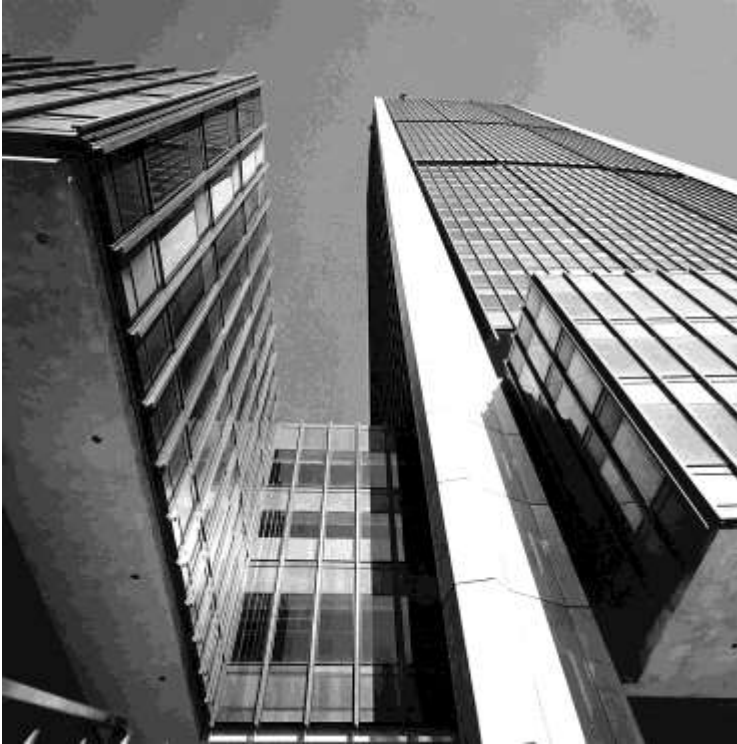
Fig. 16 View of the corner column
