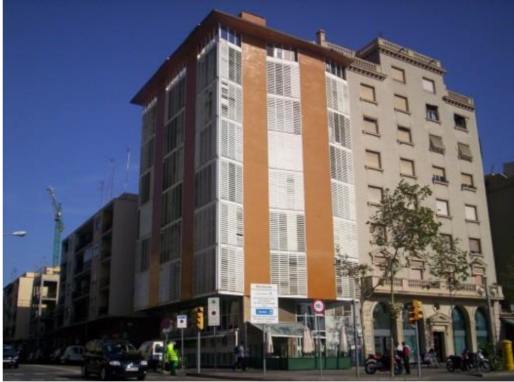
Fig. 19 LA BARCELONETTA APARTMENT BUILDING, Barcelona, 1951 Jose Antonio Coderch
