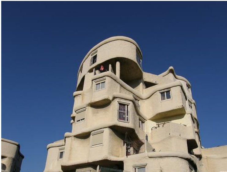
Fig. 10 HOUSING PROJECT, Angers (Maine-et-Loire) 1972-76
