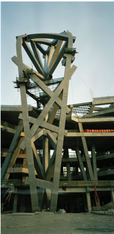
Figure 4: Truss-Column ("Olympic," 2006)
