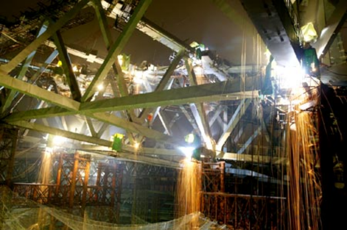
Figure 6: Workers finish welding of steel structure of the Bird's Nest (Steel, 2006)
