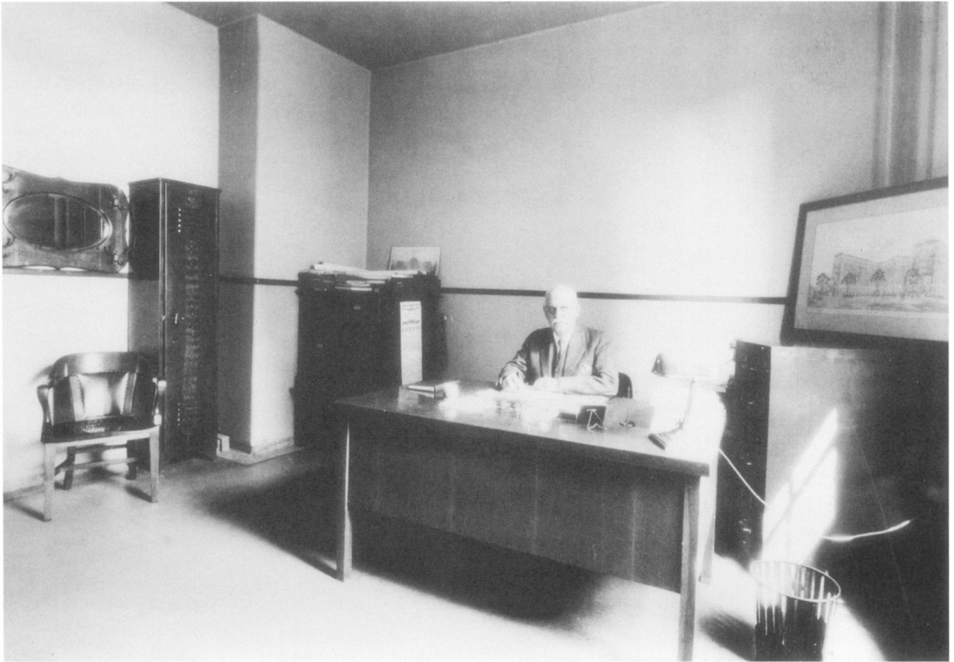
FIGURE 24: Stevens and Lee, Hôpital Notre-Dame, Montreal, about 1930, superintendent's office
