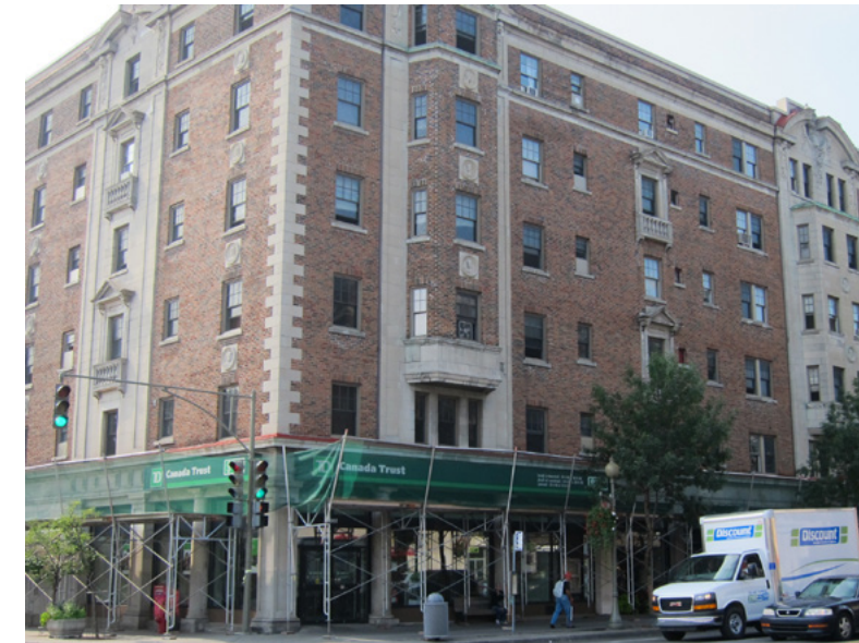
Figure 11: Scaffolding on the Pickwick Arms building
