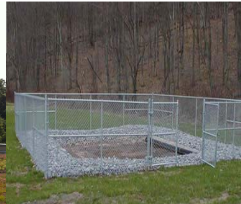
Sand filter near garages, NYC
