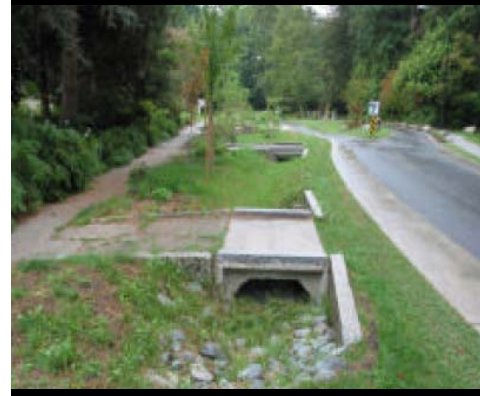
Vegetated Swale, Vancouver (Crown Street)
