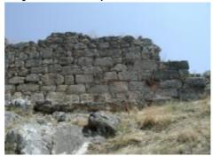
Figure 16. Mendenitsa, Isodomic ashlar reused in Outer wall.
