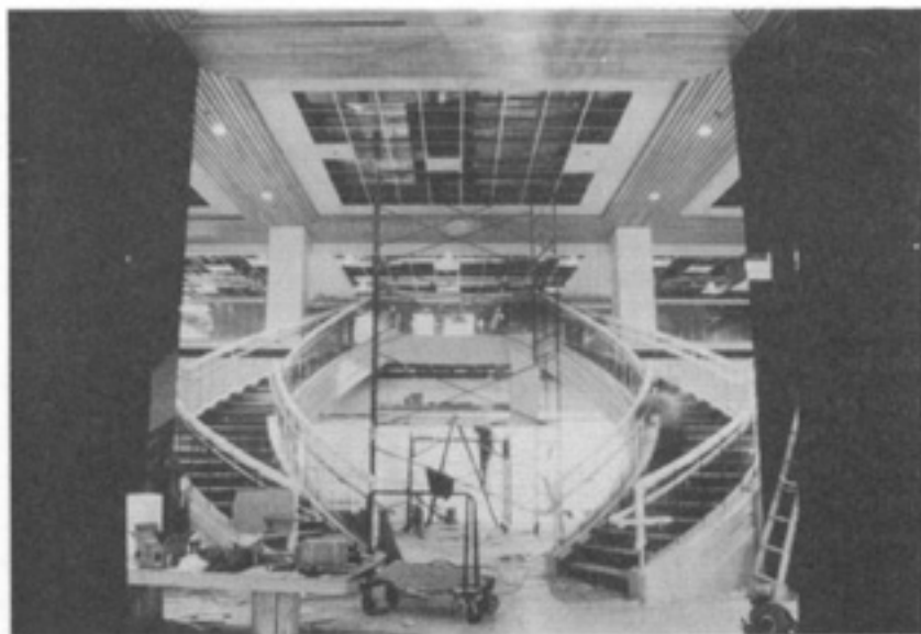
WHW Architects, Halifax Infirmary under construction, 1997 (Courtesy WHW Architects).
