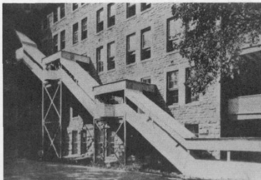
Fire chute, Grey Nuns' Military Convalescent Hospital, Montreal ( Construction , 10, 9 [September 1917]: 299).
